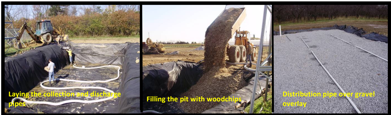
Figure 2. Construction stages of a gravity-fed bioreactor.
